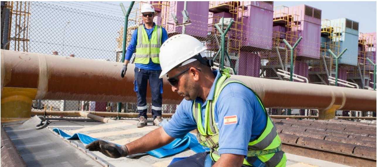
OSWS project in Oman.
