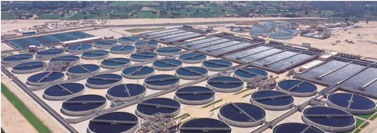
Abu Rawash wastewater treatment plant, Egypt.
