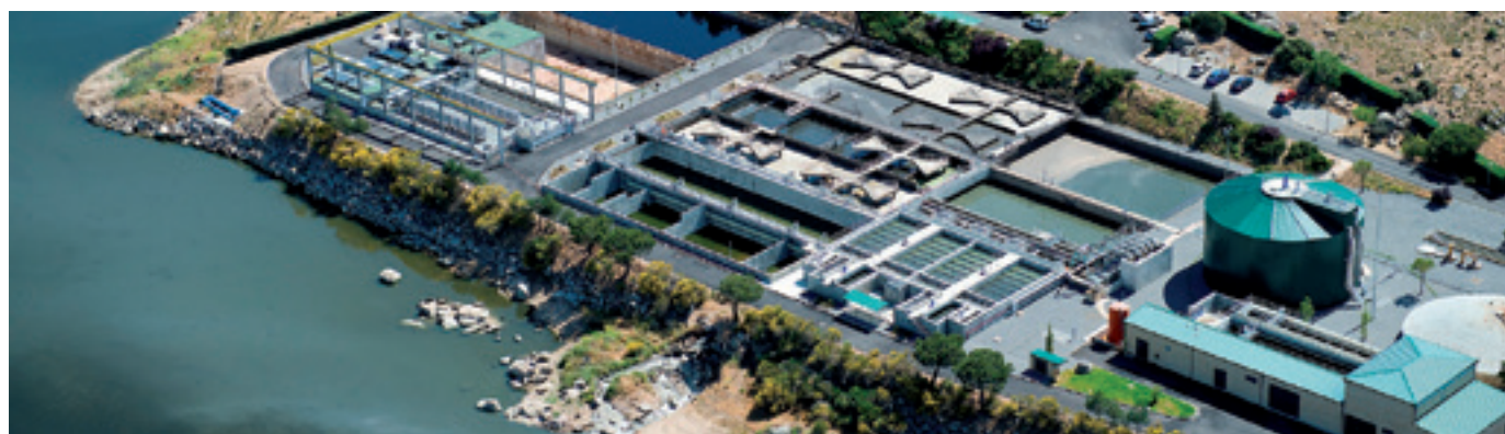
Aerial view of the WWTP in Ávila.
