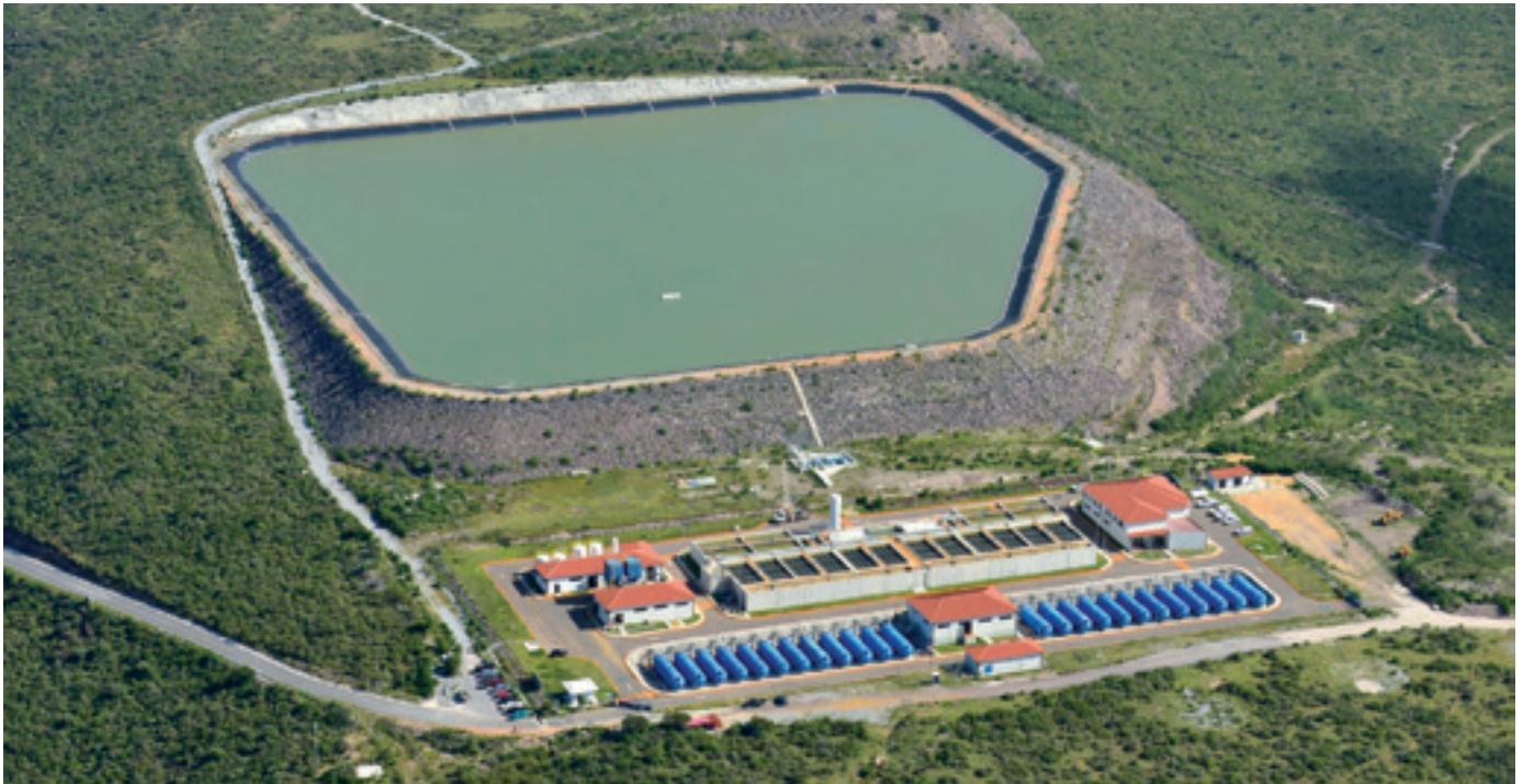
Aqueduct and Aqueduct II treatment plant, Mexico
