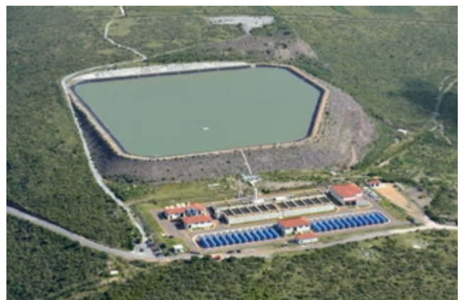
Querétaro aqueduct, Mexico.
